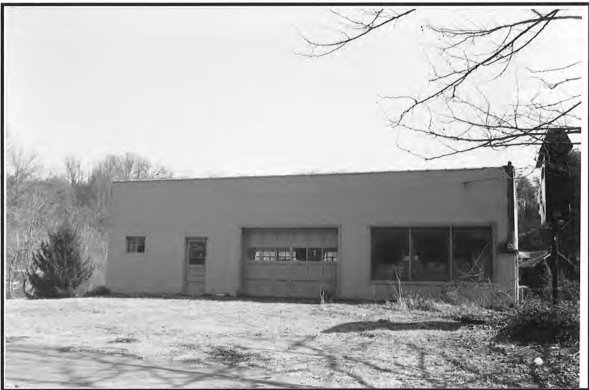
39. Commercial Building, 10 Chestnut Mountain Road
