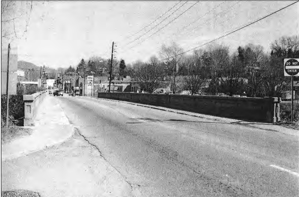
Pigeon River Bridge – view to east
