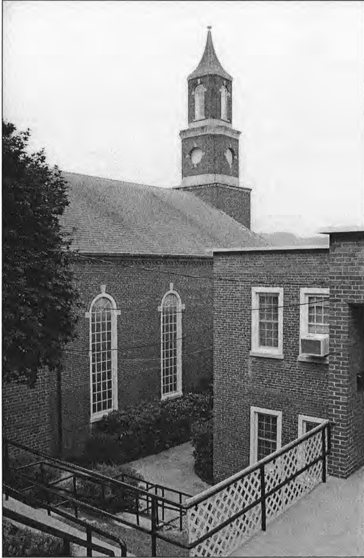
Central United Methodist Church – oblique view from SE
