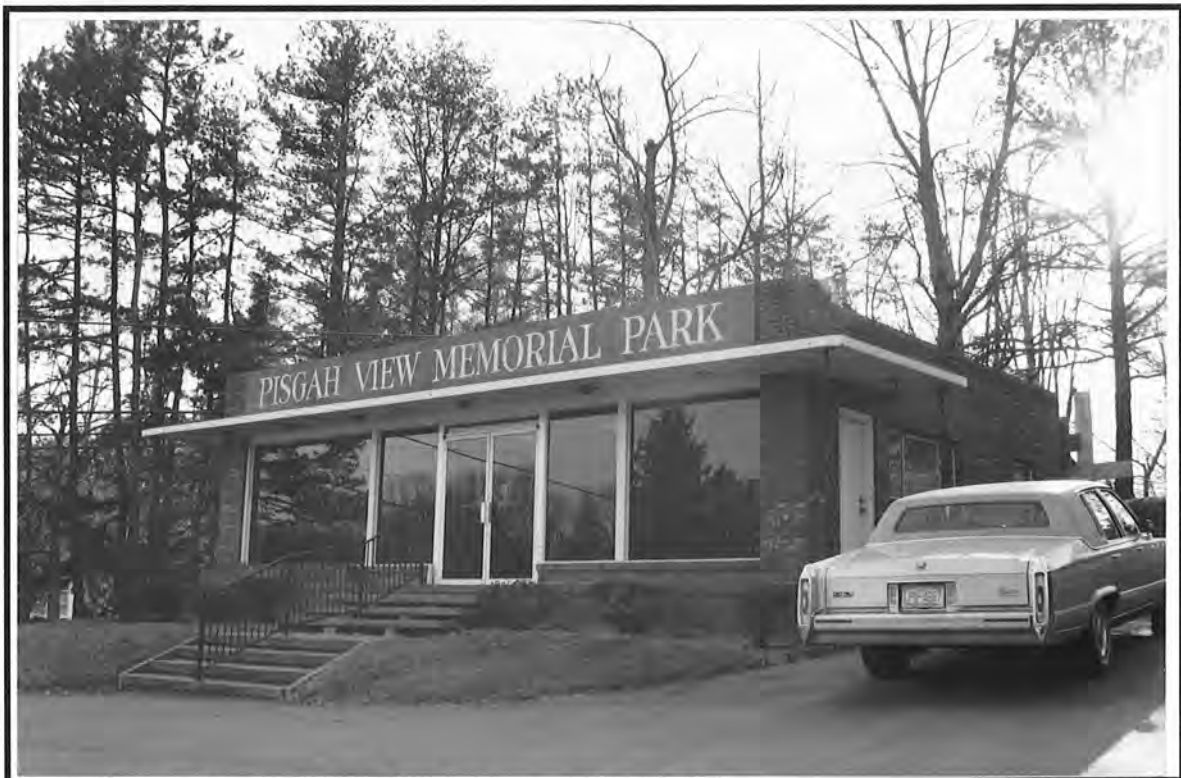
118. Pisgah View Memorial Park Office, 1529 Smokey Park Highway
