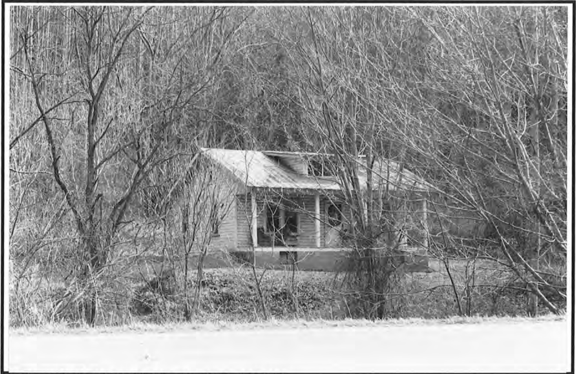
69. House, S side US 19-23, 0.3 mi E of jct w/SR 1600
