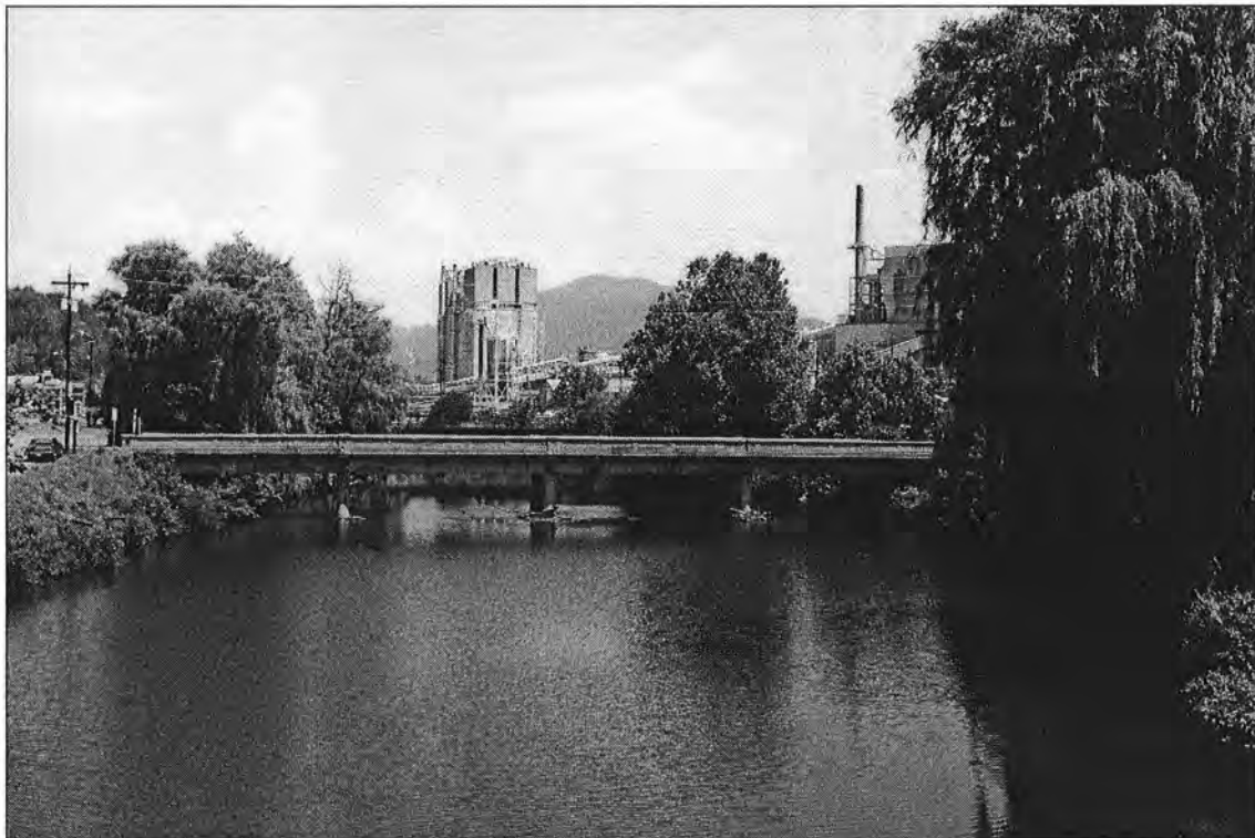
Pigeon River Bridge – view to north
