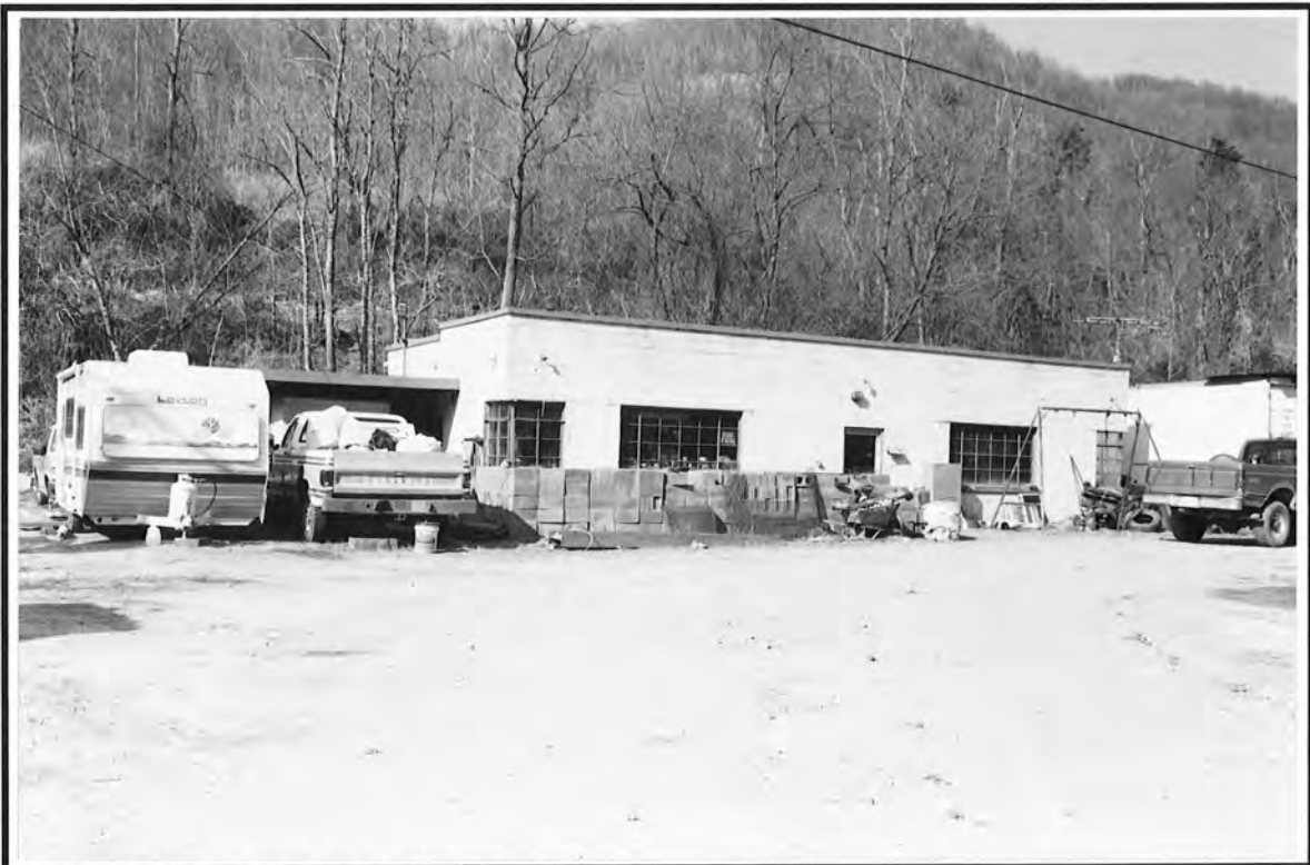
65. Commercial Building, 1190 Asheville Highway
