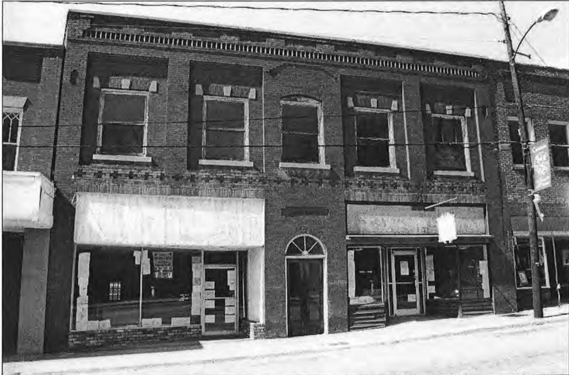
Downtown Canton Historic District – Freeman-Hudson Building (#19), 125-127 Main Street
