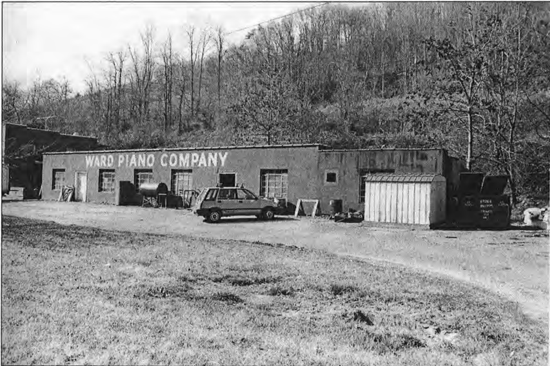
Ward Piano Company (Property #66) – oblique view from SE
