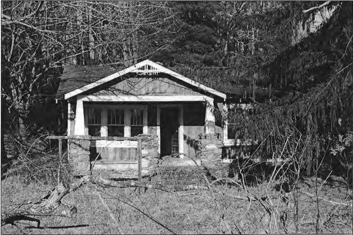
House (#100) – front (east) façade
