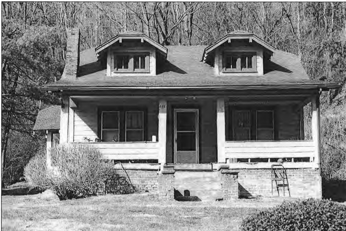
House (#58) – front (south) façade
