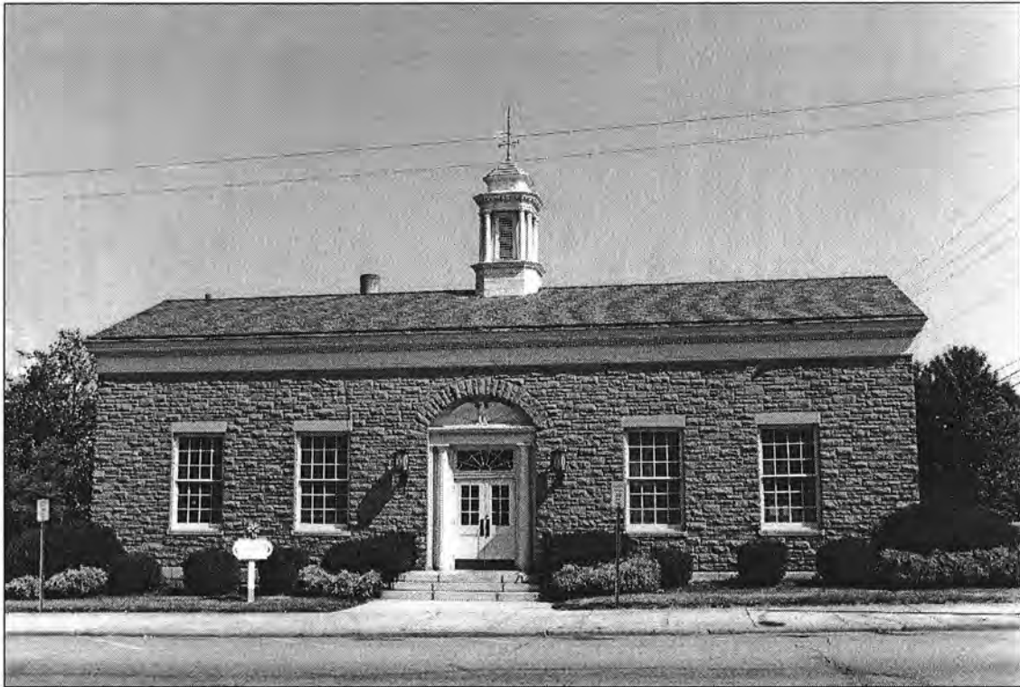
(Former) United States Post Office – front (south) facade
