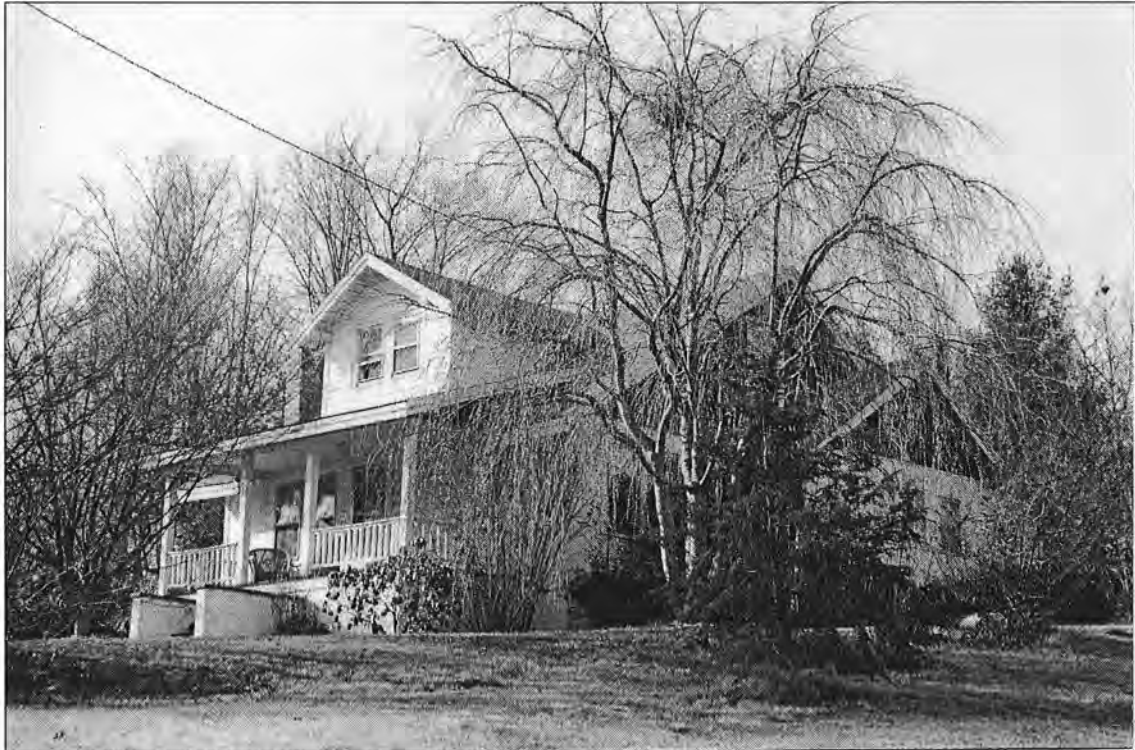
House (#99) – oblique view from SE
