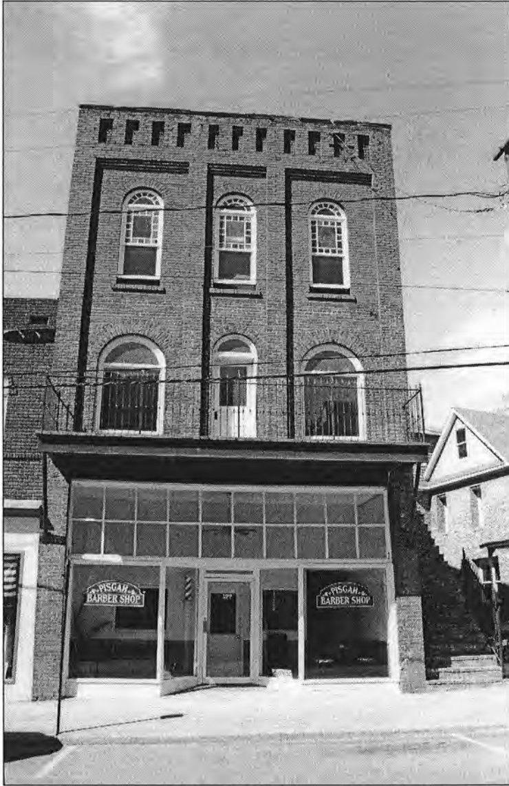
Downtown Canton Historic District – Sharp Building (#16), 109 Main Street
