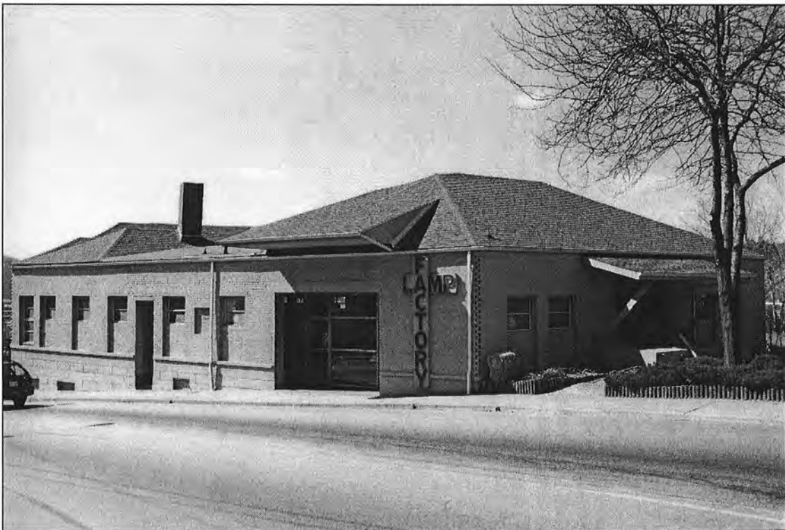
Downtown Canton Historic District – (former) Bell Motor Company (#27), 35 Church Street
