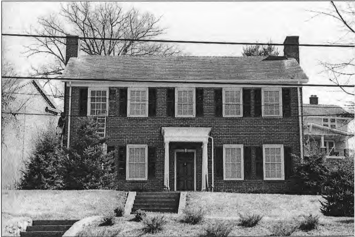
House (#26) – front (north) facade
