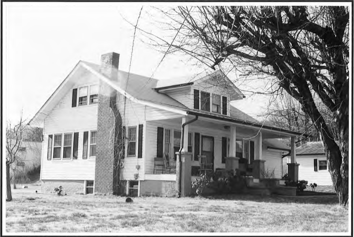
93. House, 705 North Morgan Branch Road
