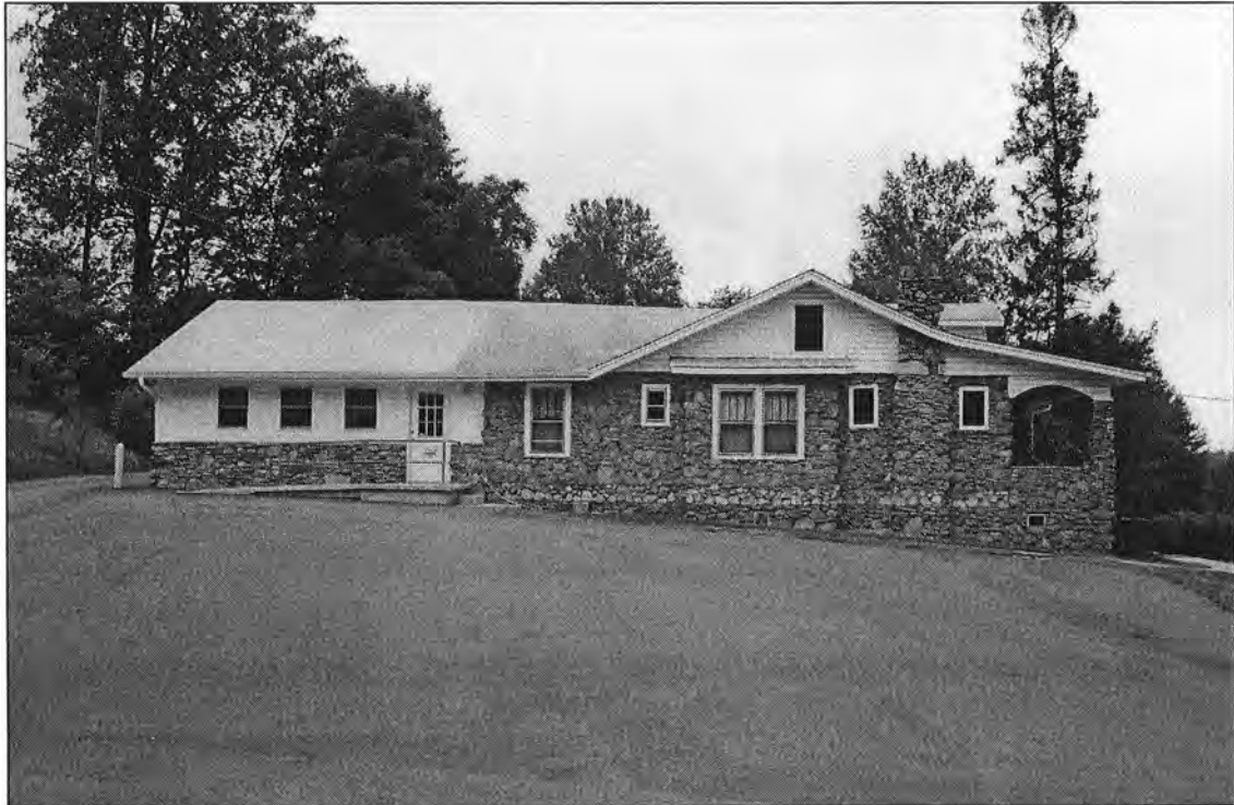
House (#116) – west side view
