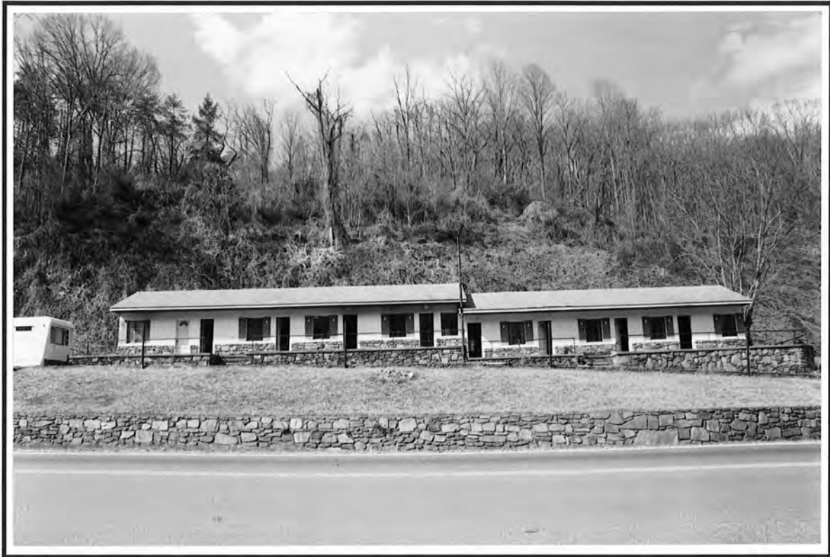
46. (former) Motel, 2710 Asheville Highway
