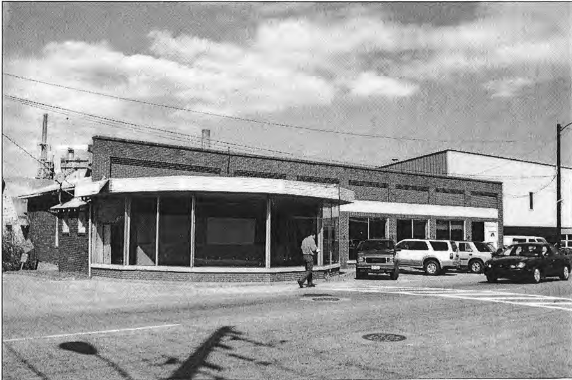
Champion Motor Company Building – oblique view to NE
