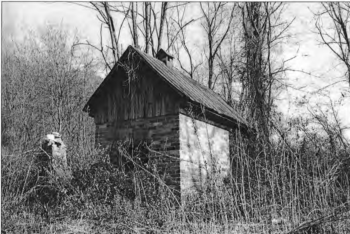
Spring house (#86) – oblique view from NW
