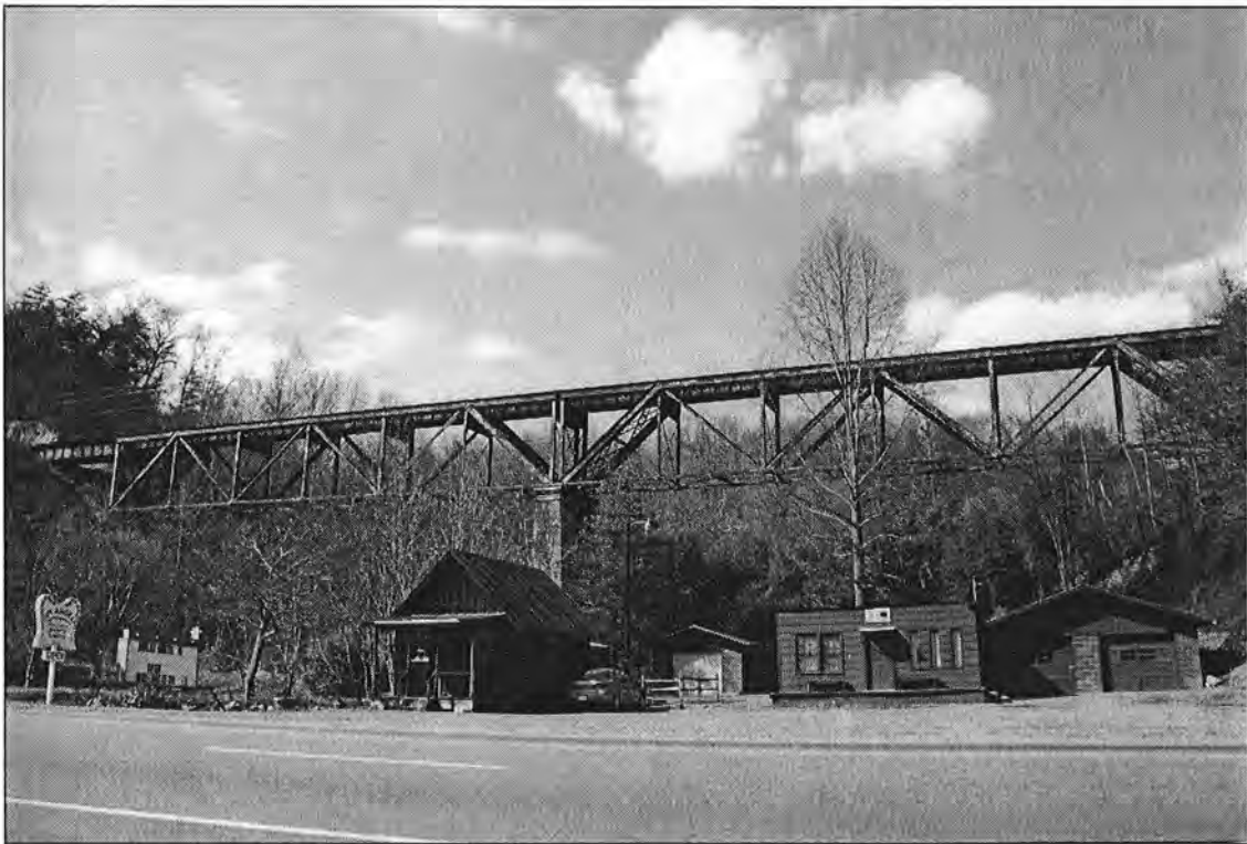
North Hominy Creek Railroad Bridge – overall view from SE
