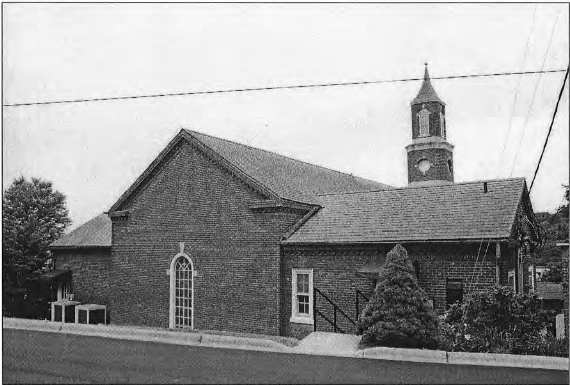
Central United Methodist Church – rear façade
