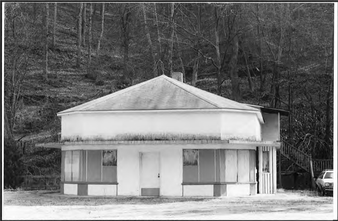
64. Commercial Building, S side US 19-23 (Asheville Highway)
