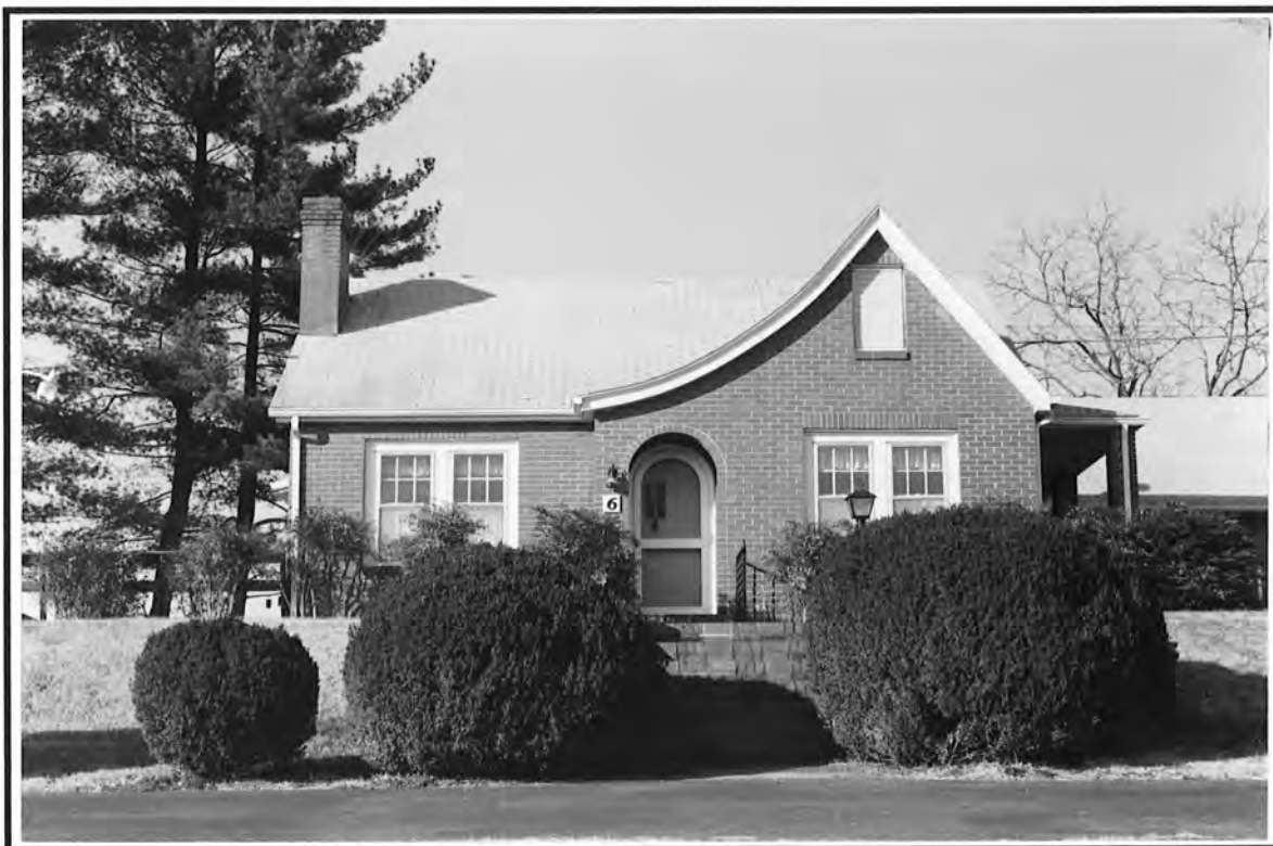
111. House, 6 Justice Ridge Road
